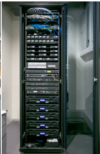
Extron presentation switchers, matrix switchers, and audio processors are at the core of AV systems installed across the THEi campus. Left: podium-mounted standard classroom AV system. Right: rack-mounted lecture theater AV system.
