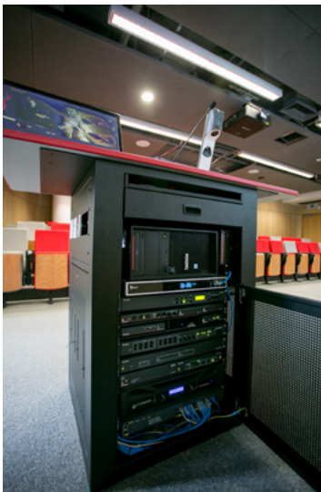
Extron presentation switchers, matrix switchers, and audio processors are at the core of AV systems installed across the THEi campus. Left: podium-mounted standard classroom AV system. Right: rack-mounted lecture theater AV system.
