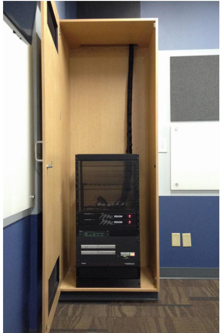
**AV switching, audio, and control equipment is rack-mounted in a cabinet that is positioned in a corner of the TEAL classroom.**
