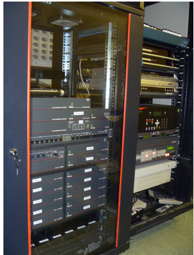
MTP DA Twisted Pair Distribution Amplifiers drive signals throughout the hall.
