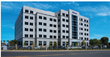
Extron USA West - Worldwide Headquarters
