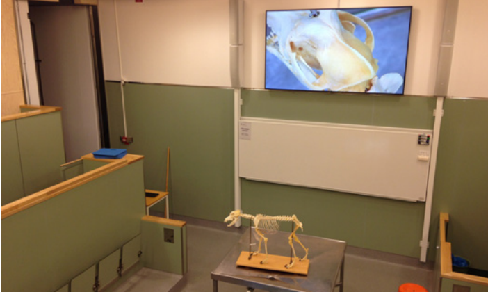
The XTP System provides complete flexibility for AV switching and distribution to the amphitheater's main display, a confidence display, as well as to systems in other teaching spaces.
